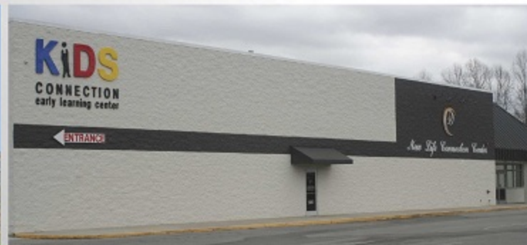
The Connection Center, home to a daycare, gymnasium, kitchen, offices, classrooms and more.
